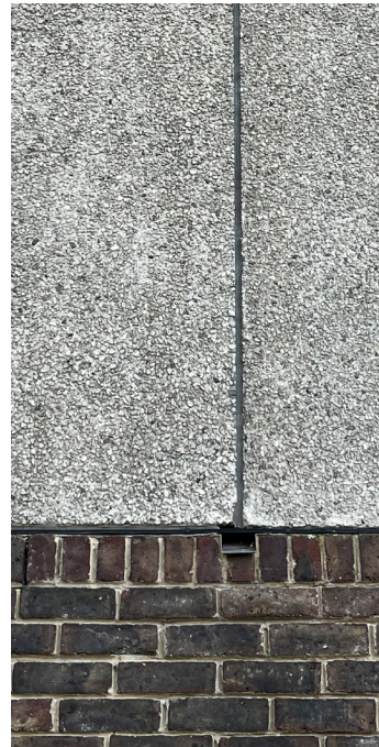
Original cavity drain to junction between precast concrete panels, 2023
