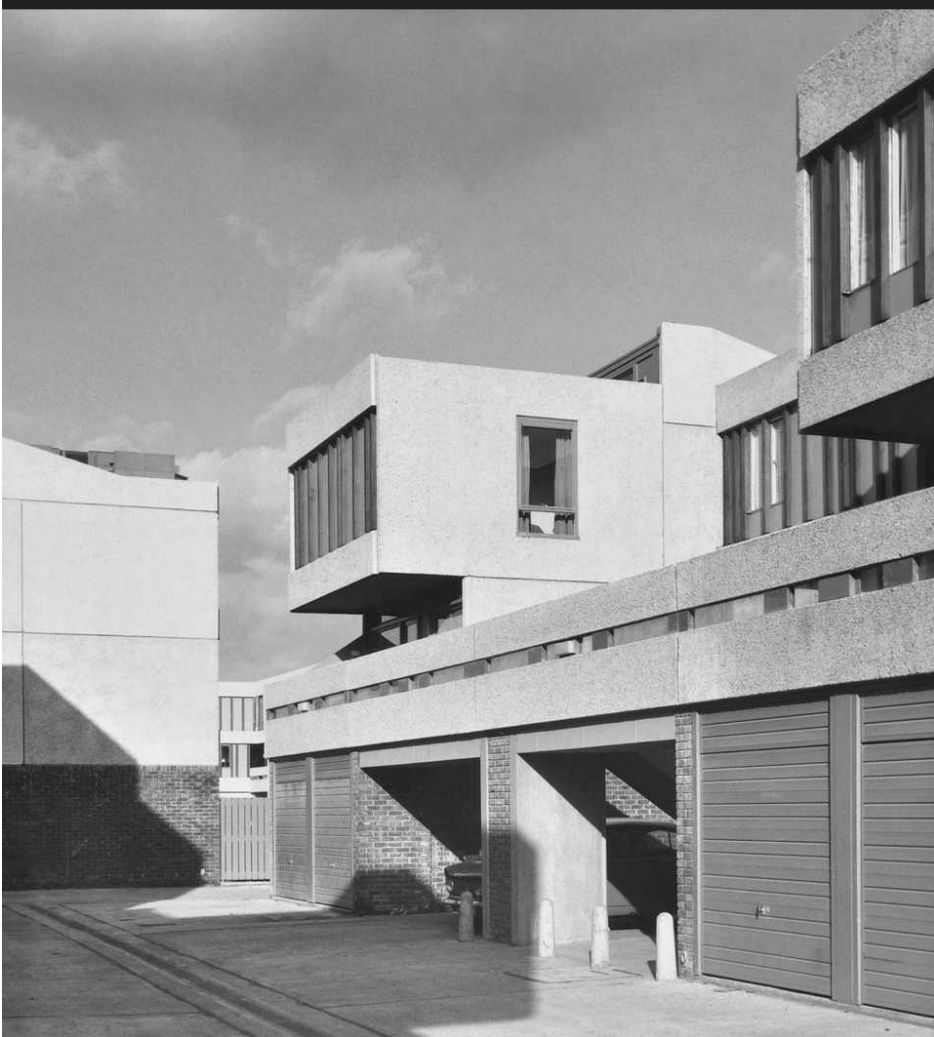
Lesnes Estate Retrofit, South Thamesmead, London
