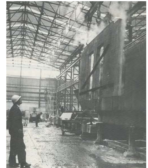
Finishing panels and removing from moulds, 1972. Copyright Peabody
