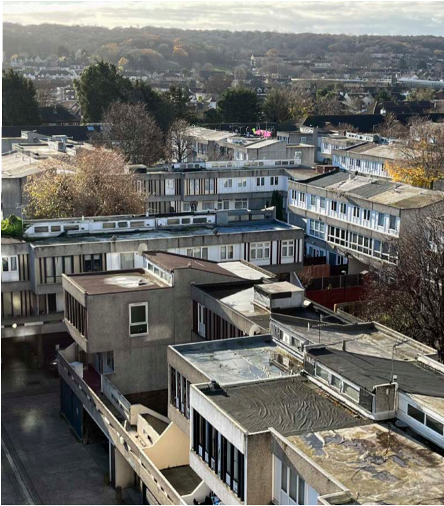
Roofscape showing varying maintenance of roofs 2023. Copyright AAB architects
