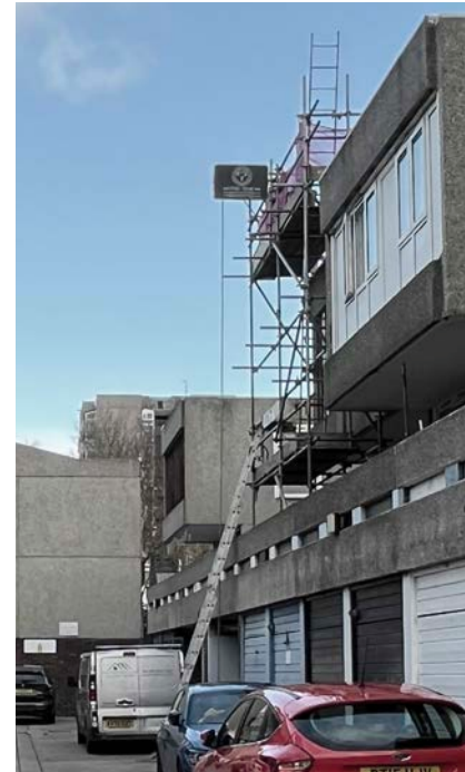
Roof repairs under way 2023. Copyright AAB architects
