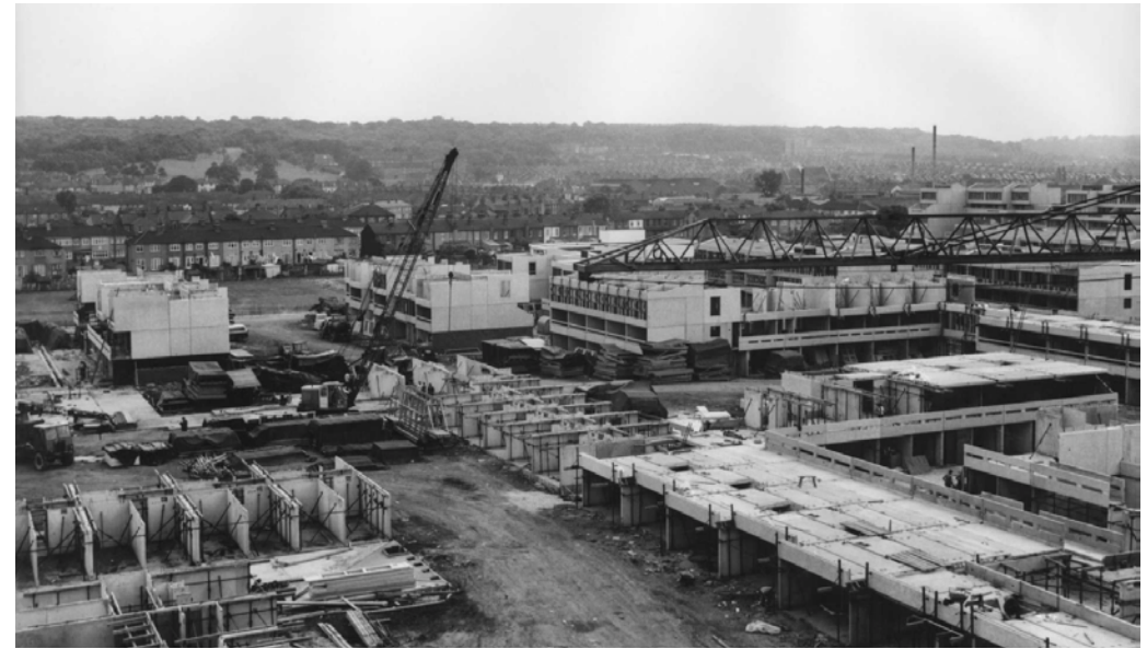
South Thamesmead under construction, 1969. Copyright Thamesmead Community Archive
